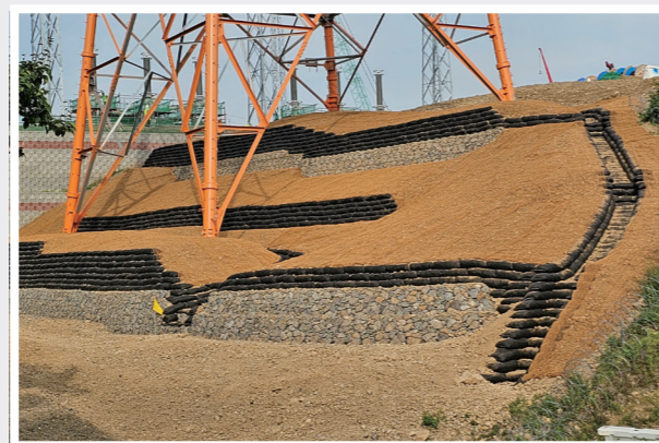
Tower foundation restoration
