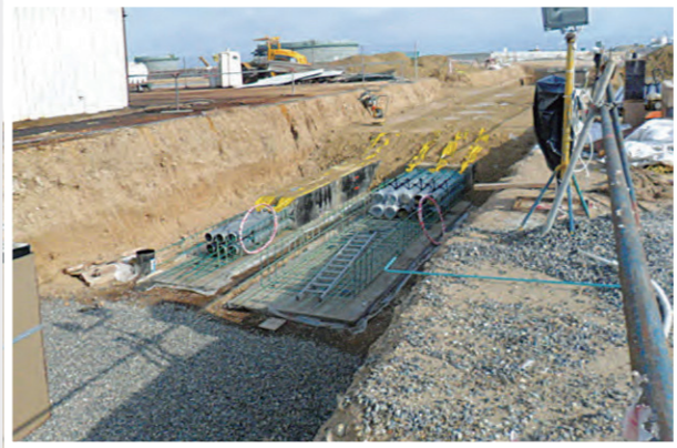
Duct Bank for HV Cable
