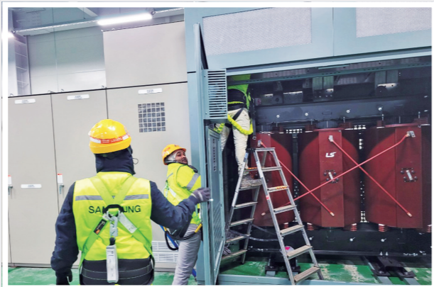
MOLD TR Installation
