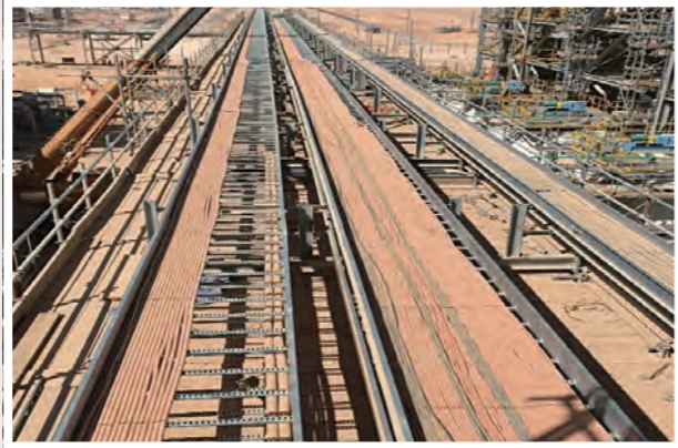
Pipe Rack Cable Pulling
