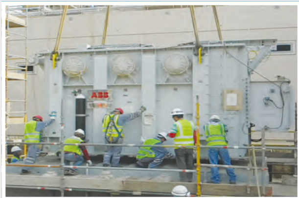
132KV Transformer Erection
