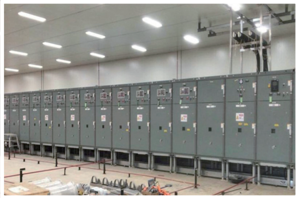
SWGR(Substation) arrangement
