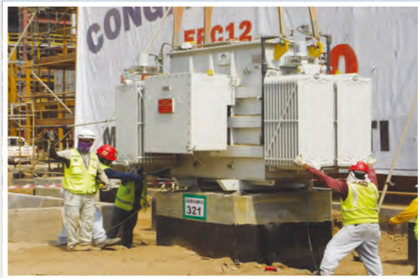
13.8KV Transformer Erection
