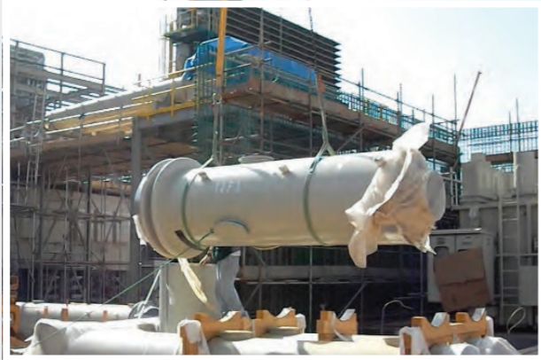
Isolated Phase Bus Duct (IPB) 3PH
