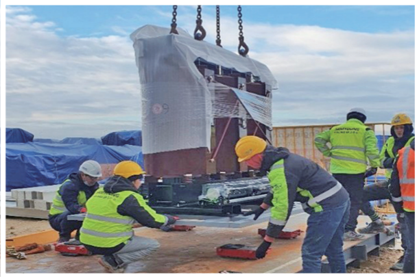
MOLD TR Installation
