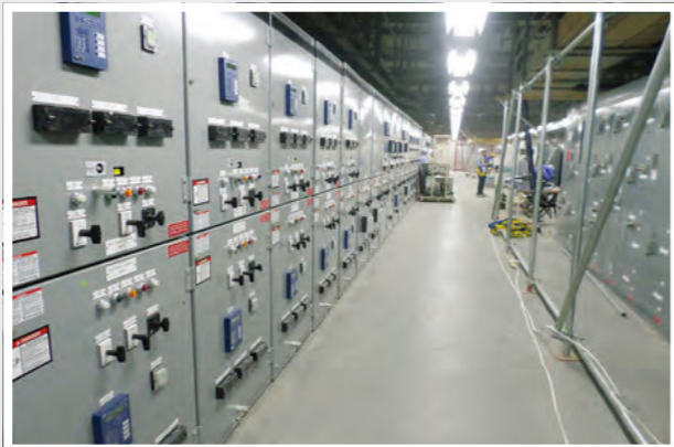
Installation of HVMV SWGR
