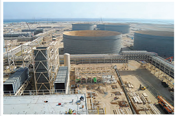
Pipe Rack For Cable Tray
