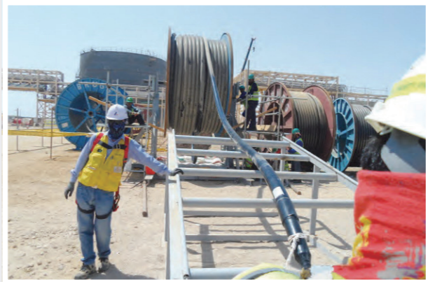
EHV Power Cable Pulling 138KV
