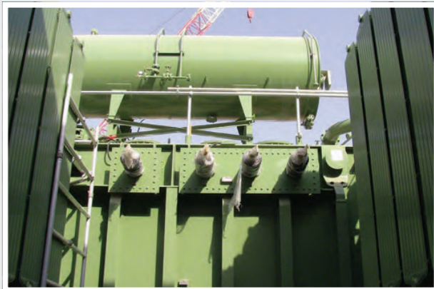
Step-Down TR, 220/33KV TR.
