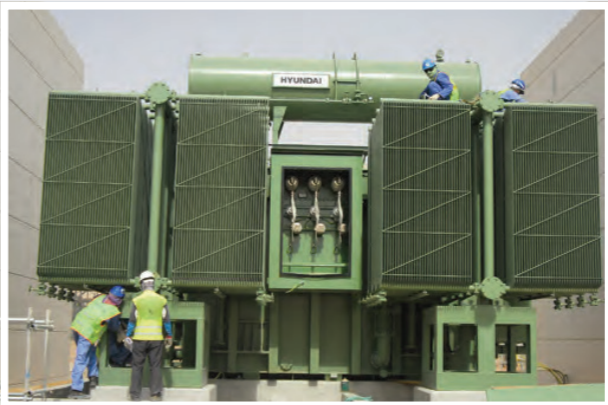
Step-Up TR, 11/230KV 40 MVA
