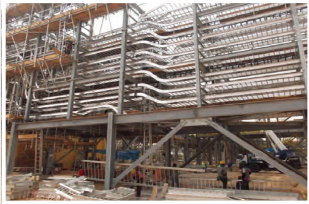
Cable Tray Installation
