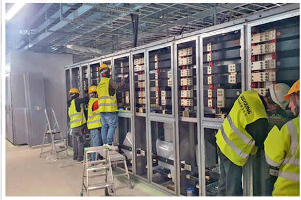
MPB LiBS SWGR Installation
