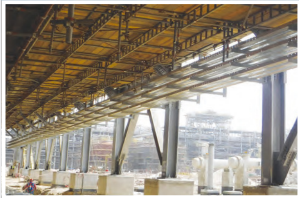
Instrument Cable Tray
