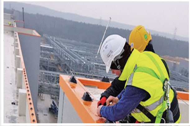
MPB Rooftop lightning wire Installation
