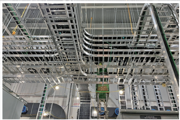
Cable Tray Installtion
