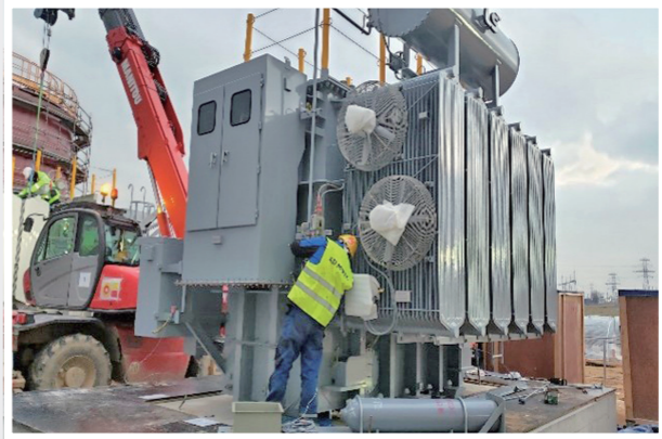
Oil-Transformer Installation
