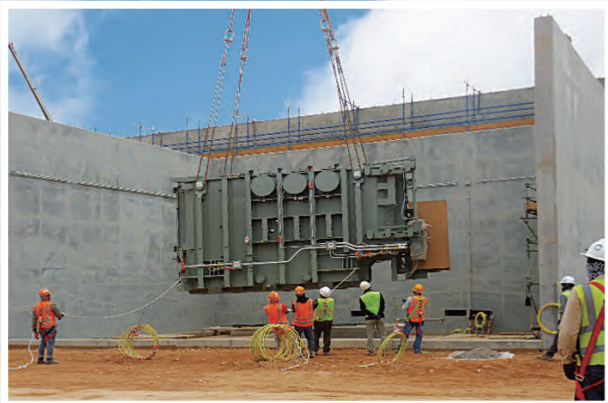
132kV Transformer Rigging
