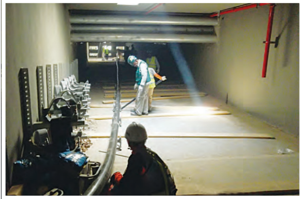
33KV Power Cable 1C-630sq
