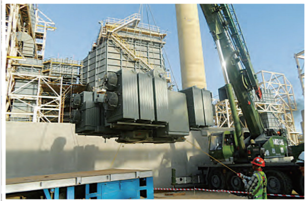
Transformer Rigging
