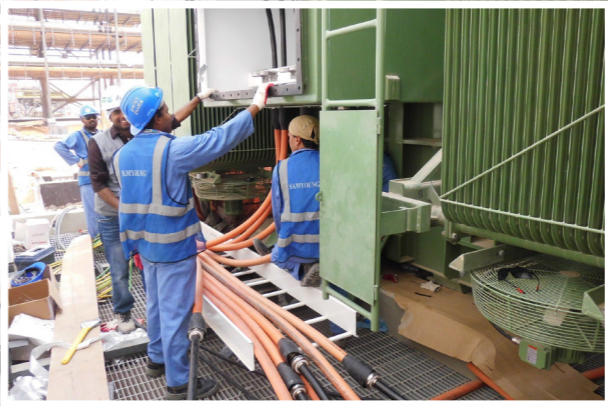
HV Cable Termination
