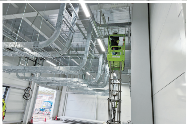
Raceway Installtion
