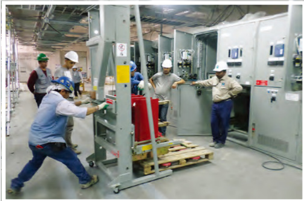
Installation of HV SWGR
