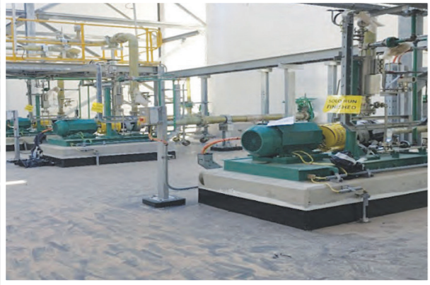
Motor Solo-run Test
