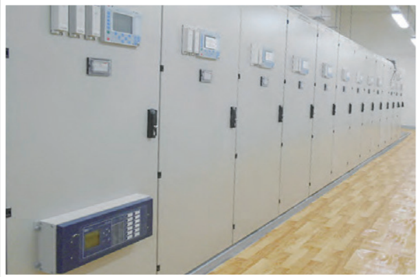
132kV SWGR Installation
