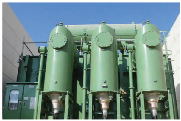
Auxiliary Transformer 13.8/6.9KV
