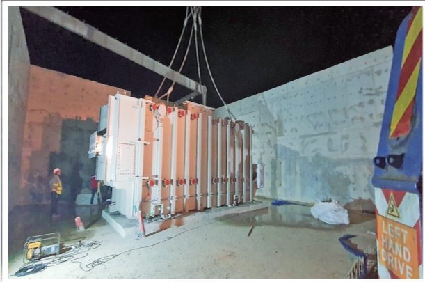
Transformer Erection
