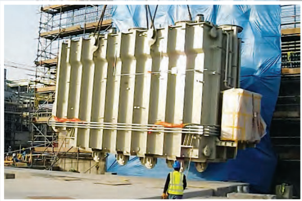
Step-up Transformer 380/13.8-18KV
