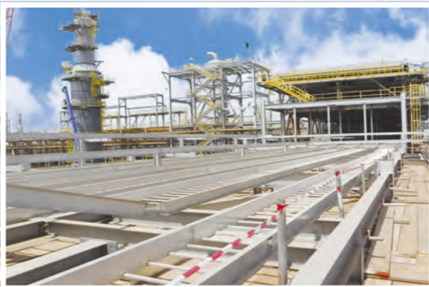
Cable Tray at Pipe Rack
