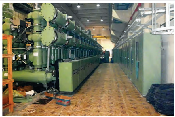
Gas Insulated SWGR Incoming Feeder 2,500A
