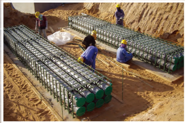
Duct Bank for HV Cable
