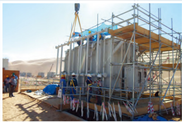
Assembling of Transformer 80MVA
