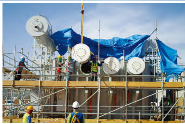
Assembling of Transformer 80-120MVA
