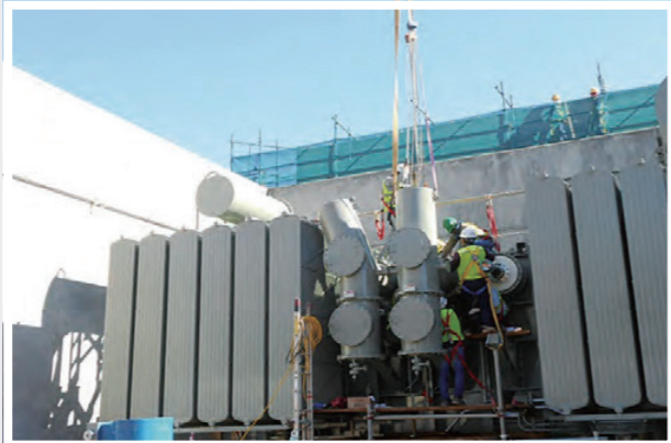
132kV Transformer Erection
